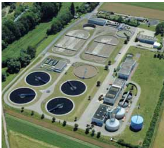
A bird's eye view of the Gotha sewage treatment plant in the state of Thüringen
