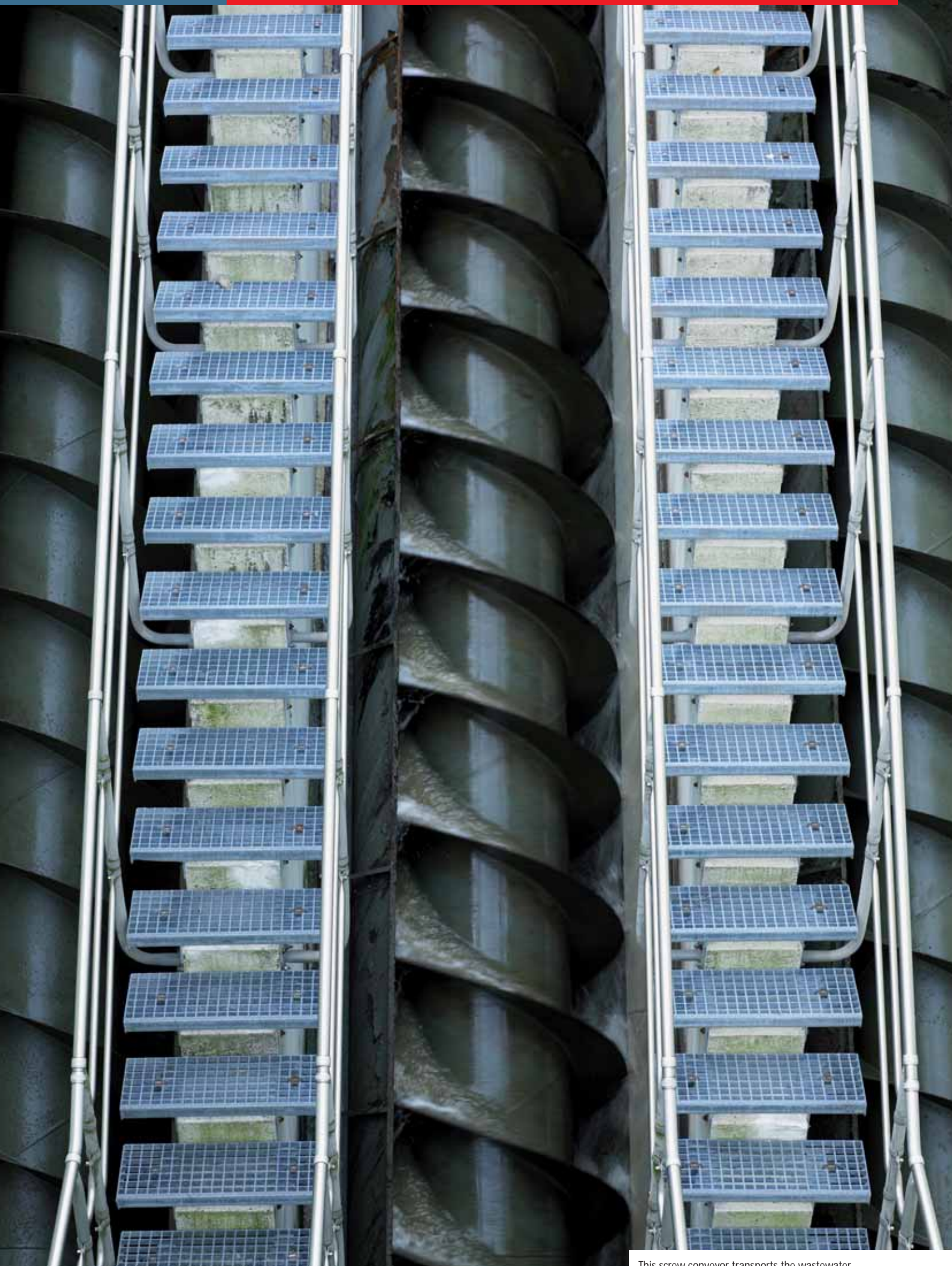
This screw conveyor transports the wastewater.
