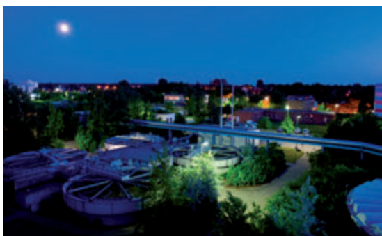
Sewage treatment plant, waterworks
