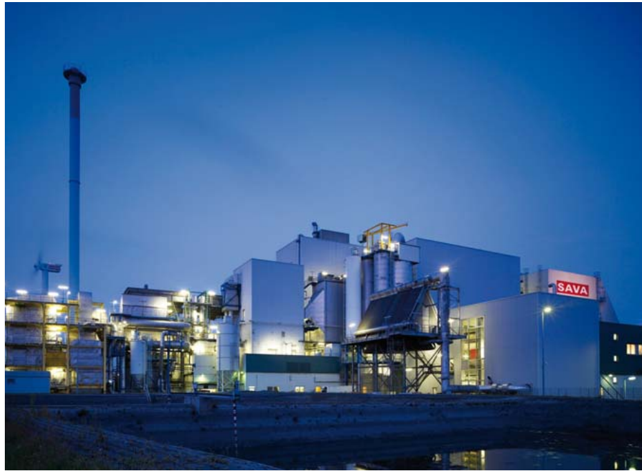
Fossil fuels are not needed during the waste incineration process. On the contrary, SAVA feeds 5,680 MWh of electricity into the national grid thus contributing towards the 'energy turnaround'
