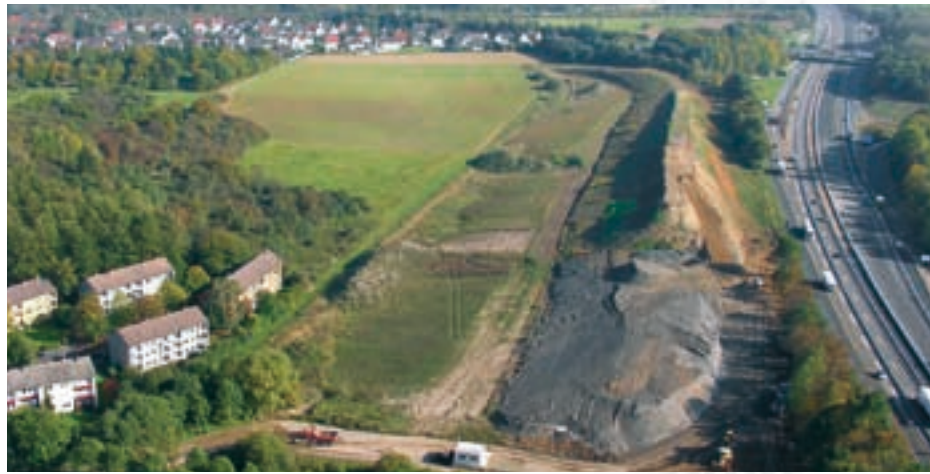
An aerial photo of the earth wall along the A44 motorway near Kassel-Mattenberg during the construction phase.
