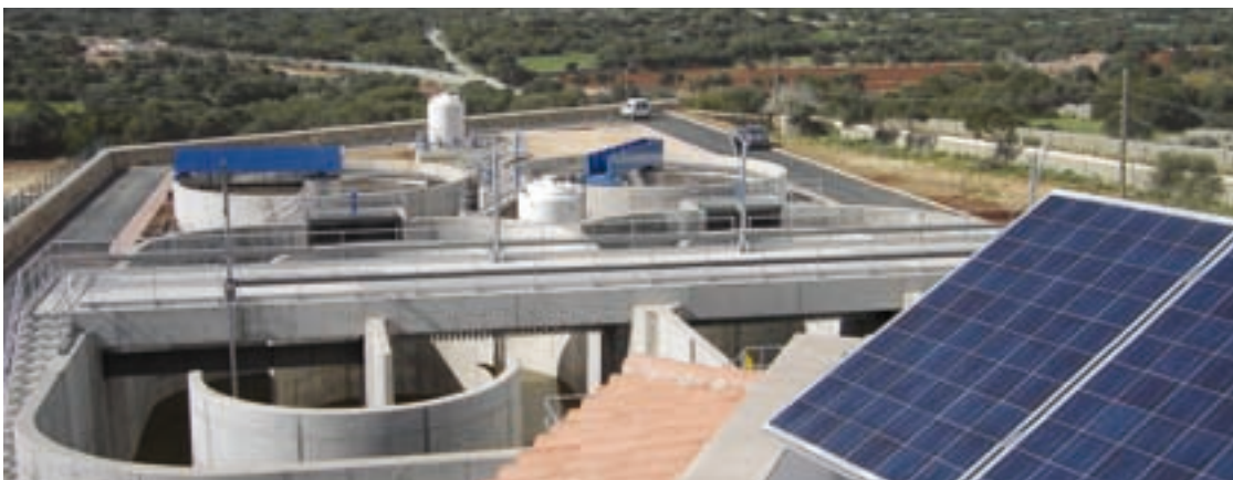
Cal en Porter, one of OMS' modern water processing plants in Spain.
